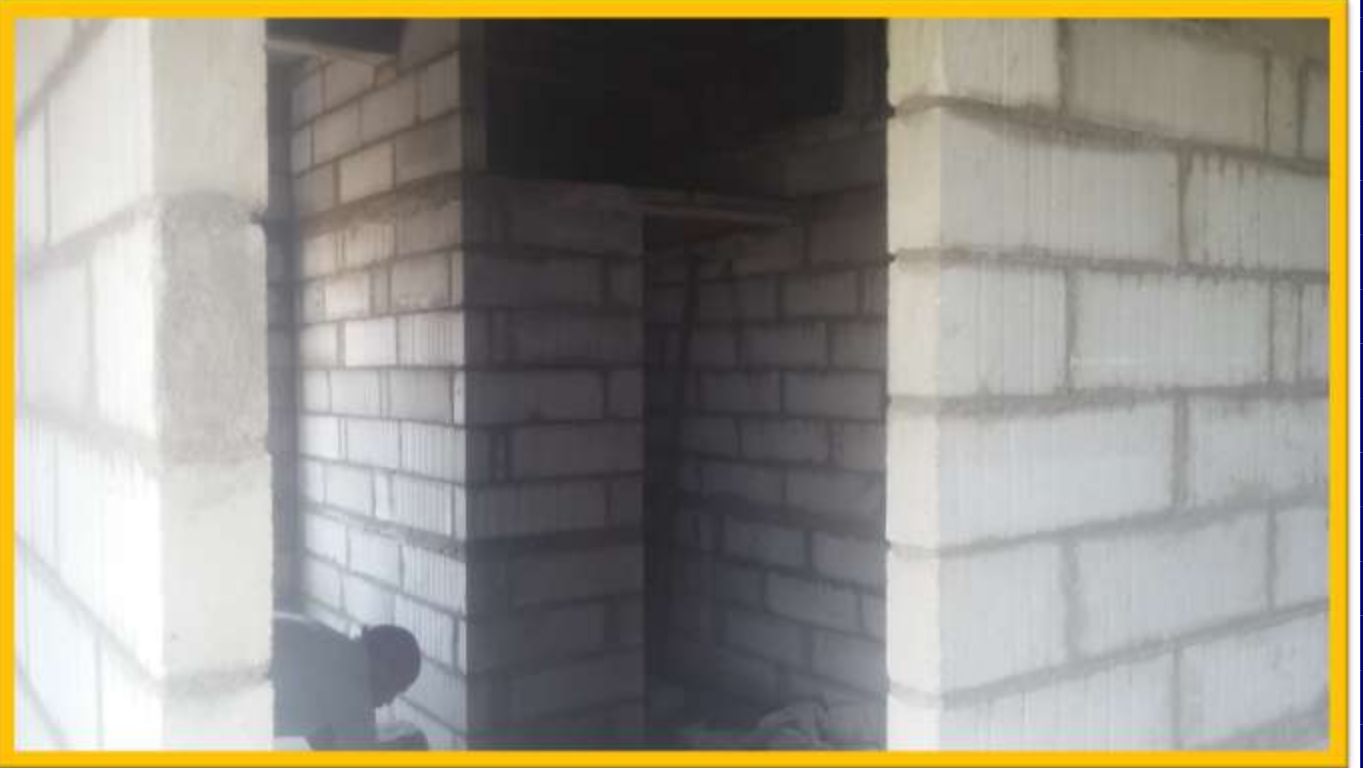
5 TH FLOOR BRICK WORK
