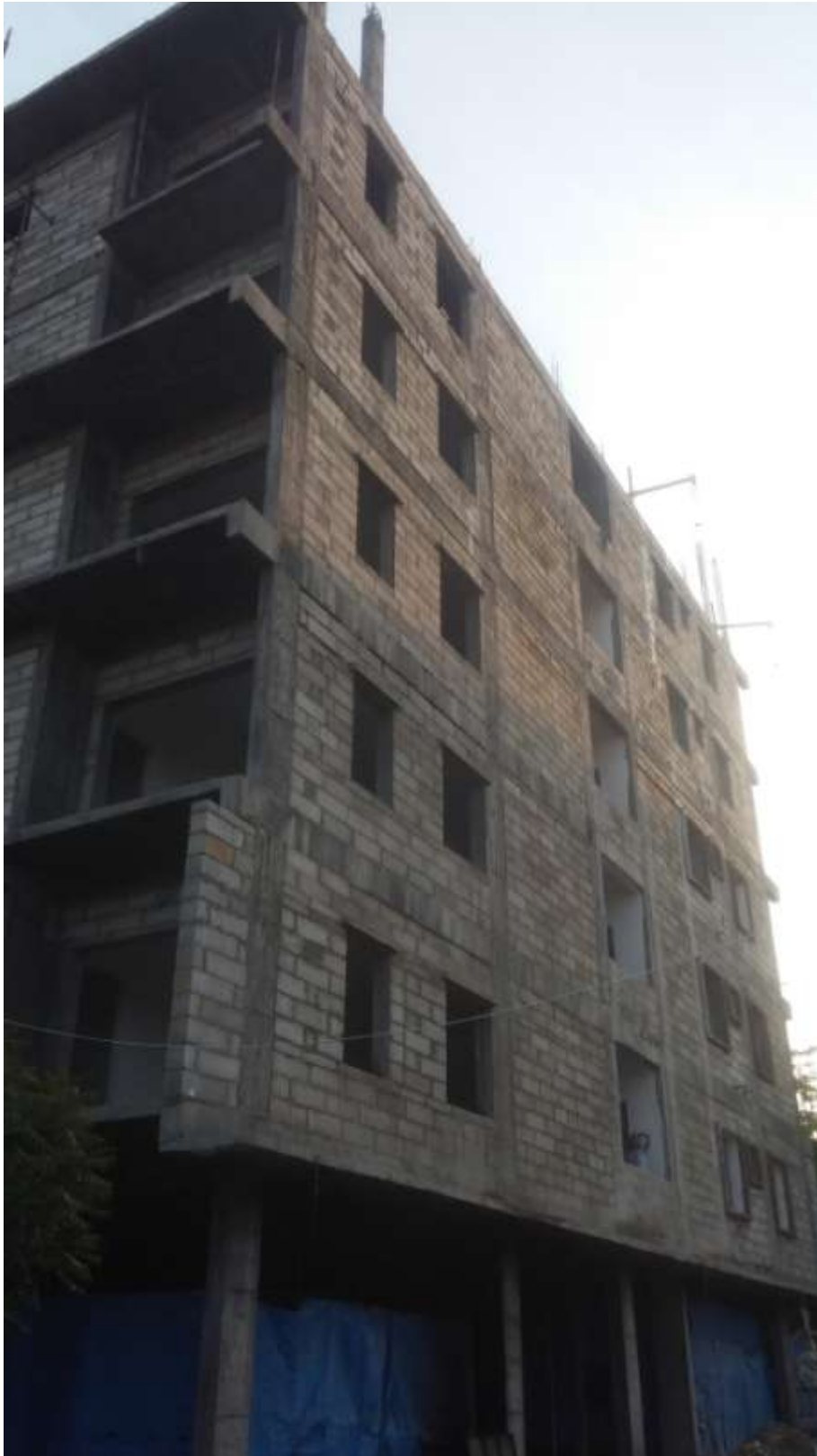
NORTH SIDE ELEVATION BRICK WORK
