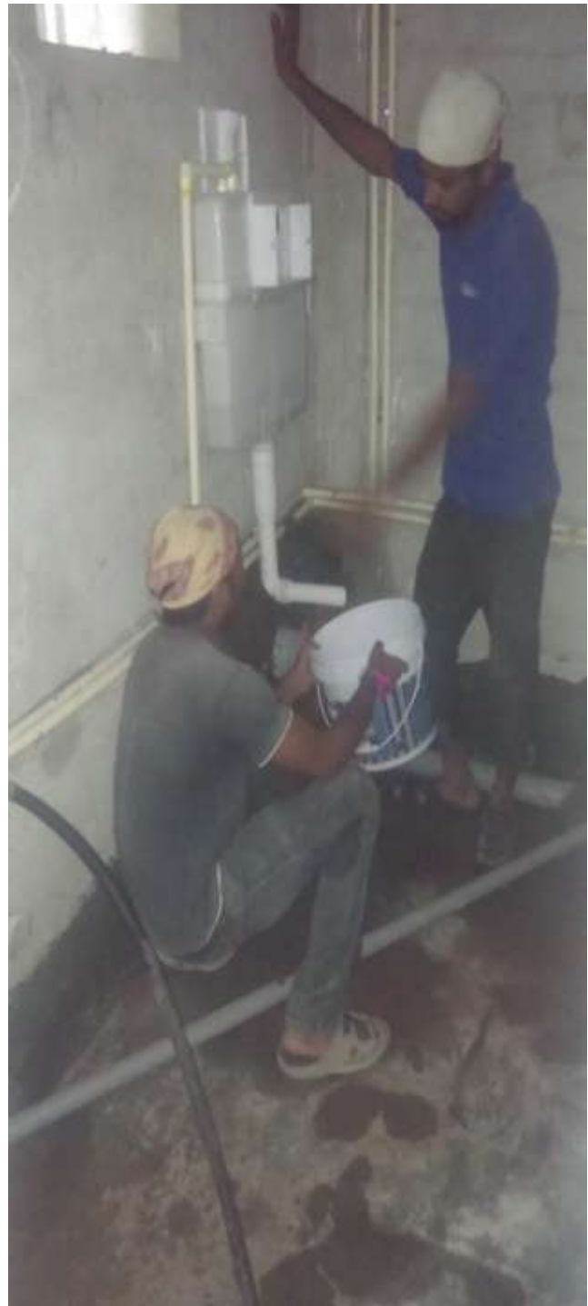
INTERNAL CPVC PIPE LINE LECKAGE CHECKING WORK
