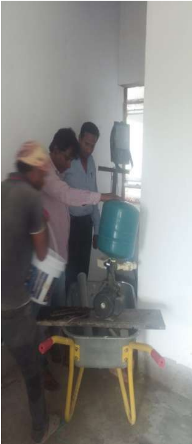
INTERNAL CPVC PIPE LINE LECKAGE CHECKING WORK
