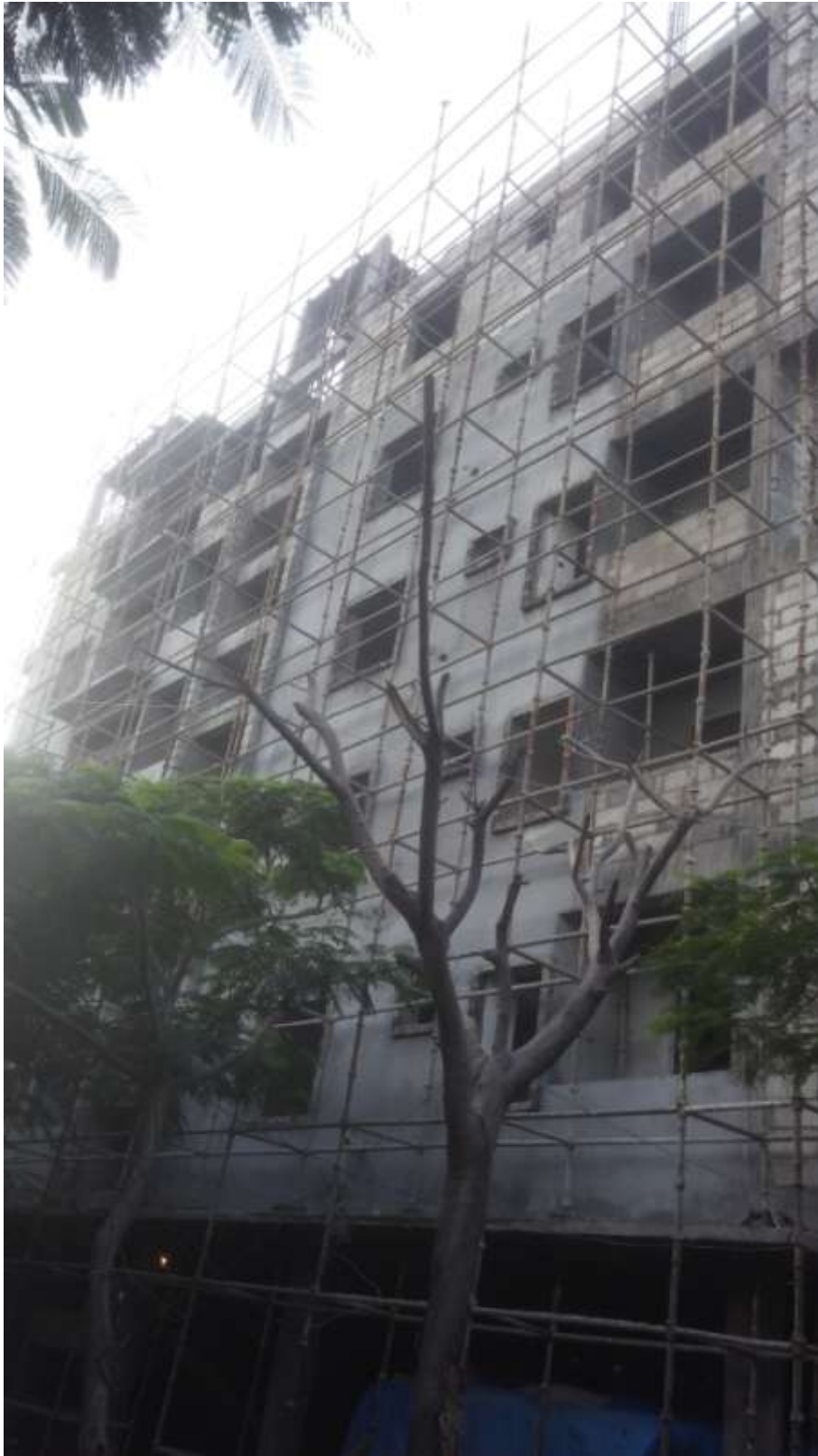
SOUTH SIDE ELEVATION BRICK WORK
