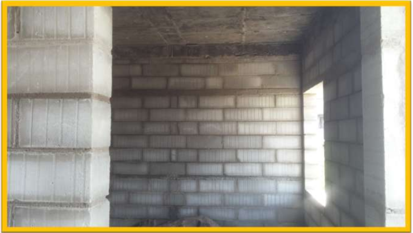
5 TH FLOOR BRICK WORK
