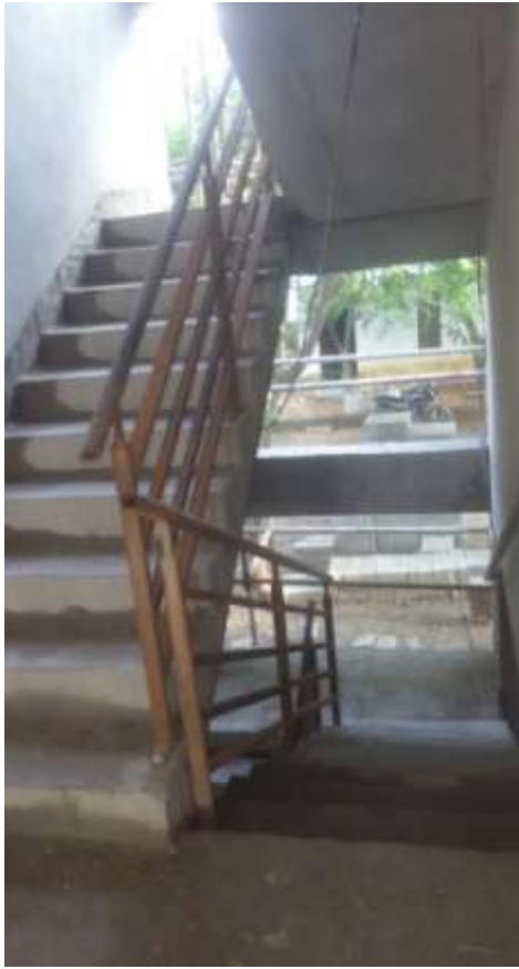
M.S. RAINING WORK ABOVE STAIRCASE WORK
