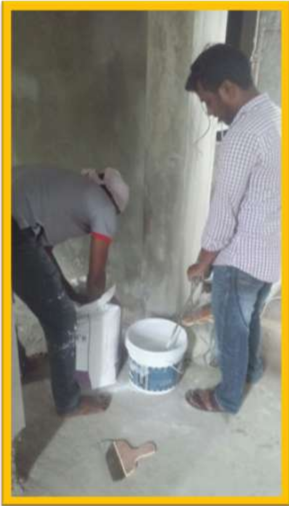
LUPPUM MIXING & LAYING WORK FOR FOURTH FLOOR INTERNAL PURPOSE.
