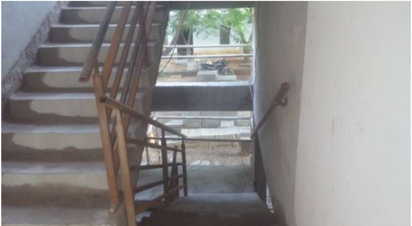
M.S. RAINING WORK ABOVE STAIRCASE WORK
