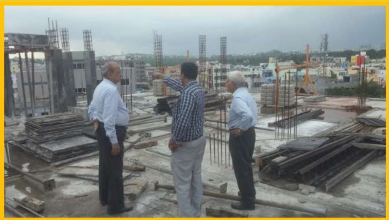
CHAIRMAN SIR SITE INSPECTION PERGOLA COLUMNS CONCRETE WORK
