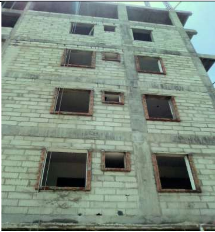
External Elevation work
