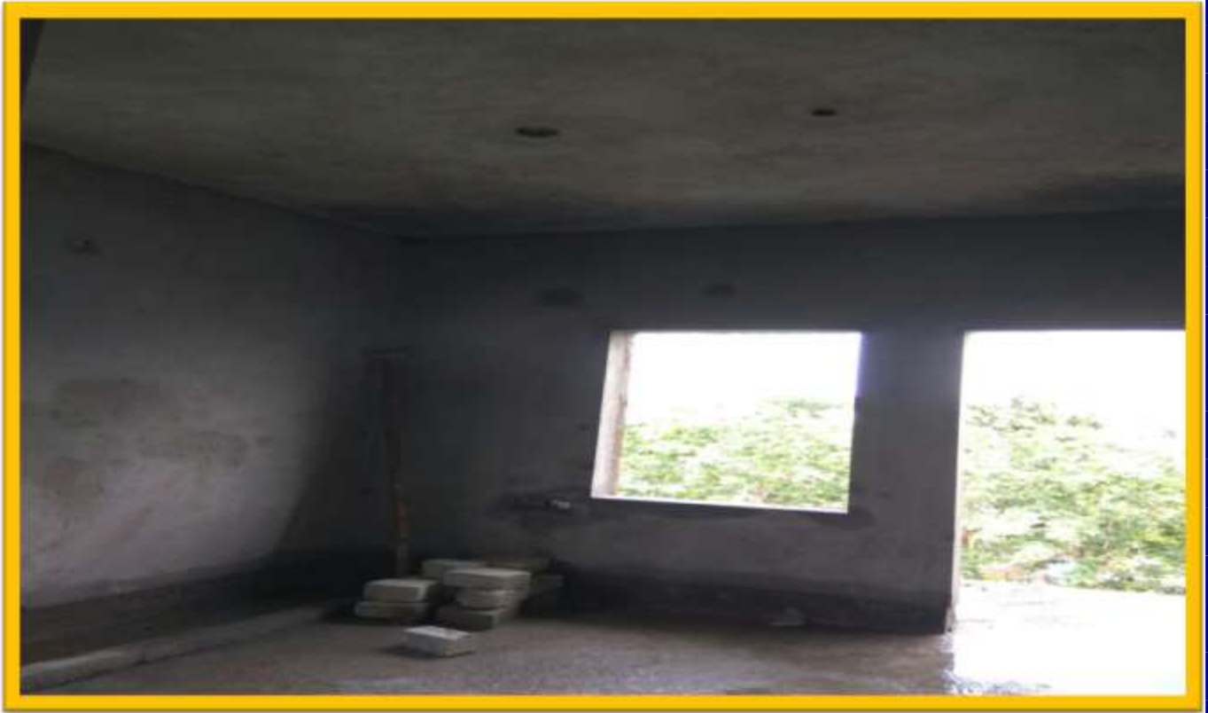
Fourth Floor Internal Plastering work
