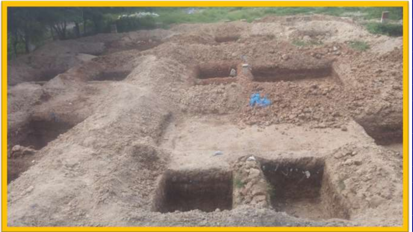
Footing Pits Excavation work
